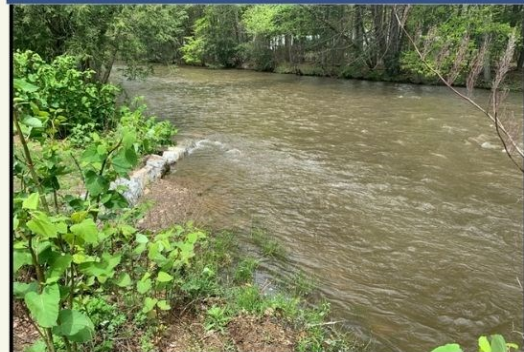
Above: Upstream rock vane
