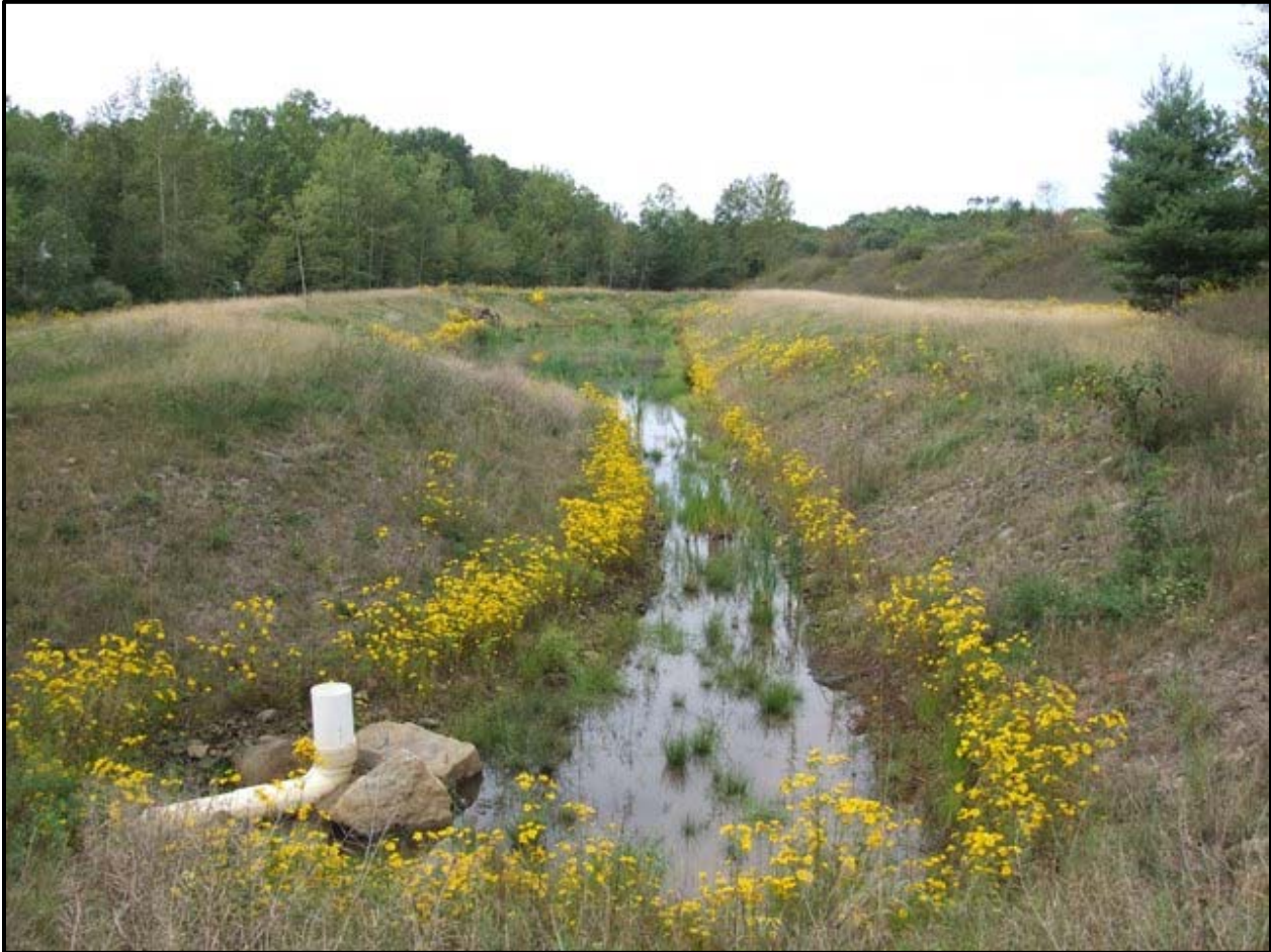
Bell Colliery Phase II Limestone Treatment Cells' Flush Water Holding Pond
