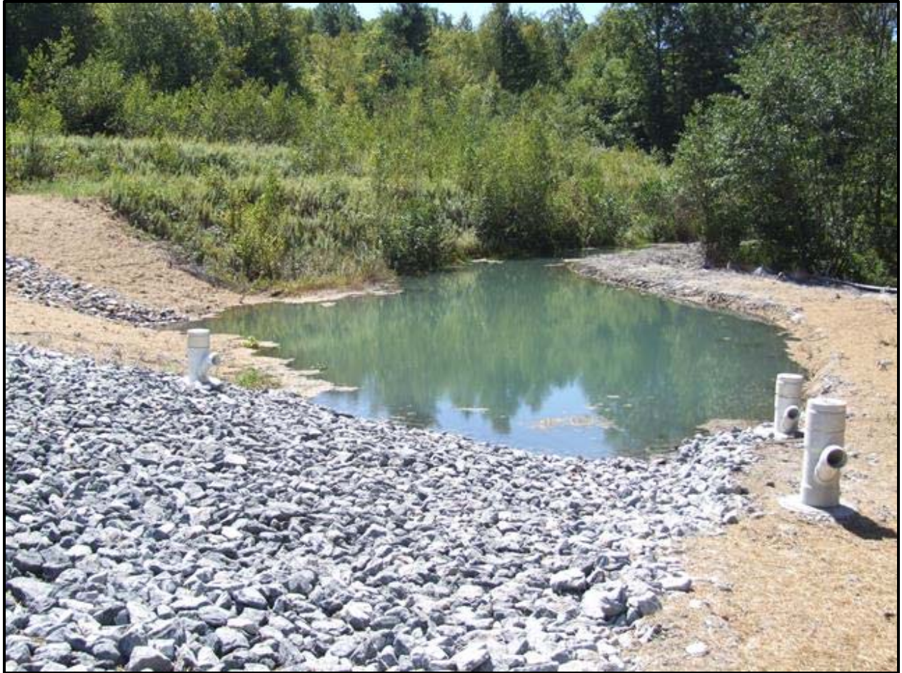
Bell Colliery Phase III Completed Aerobic Wetland
