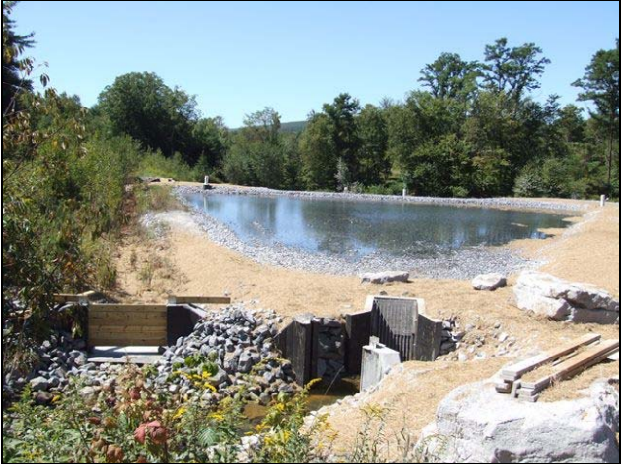
Bell Colliery Phase III Single Large Up Flow Limestone Treatment Cell
