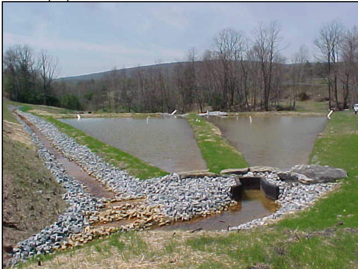
Original Bell Colliery Treatment System Down-Flow Limestone Cells
