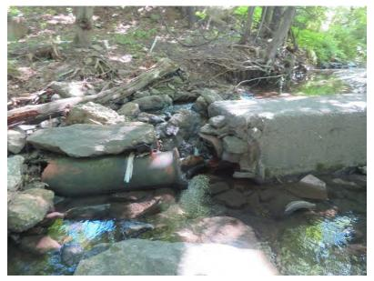
This stream segment is directly downstream of a Natural Resources Conservation Service (NRCS) riprap project. Banks are heavily eroding and as steep as 6' high in parts of this stream segment. There is a concrete encased abandoned sewer line obstructing the stream in this segment. There an existing manhole adjacent to the stream, and streambanks are eroded 3-4' high near the obstruction. Several stormwater drainage pipes discharge into this segment of the stream.
